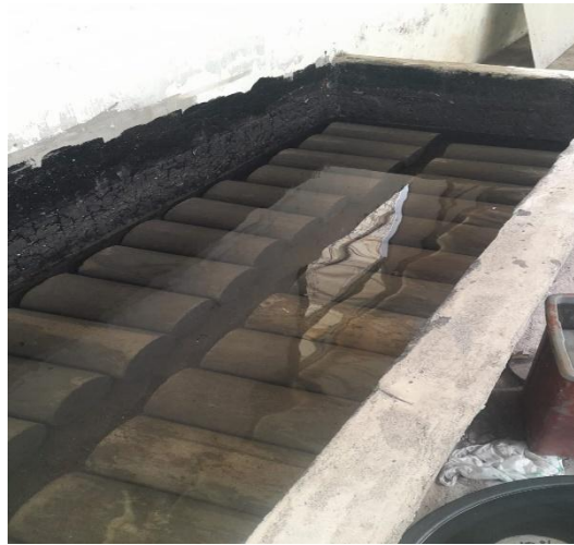
Gambar 2. Proses perawatan beton (curing)
