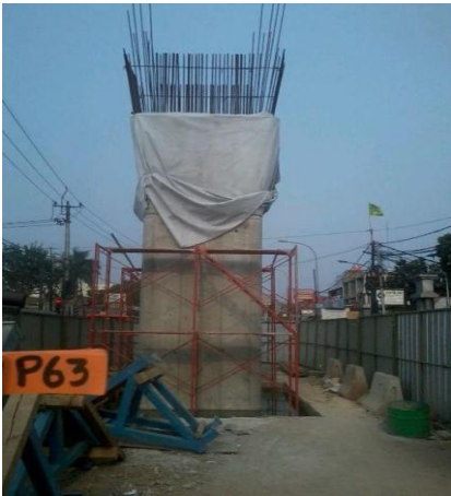
Gambar 12. Curing Beton
