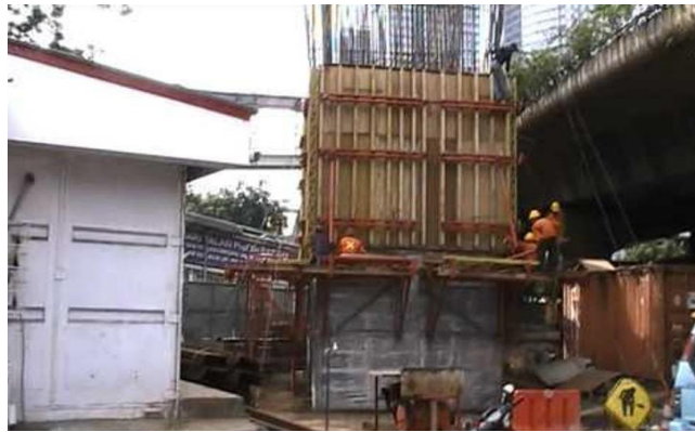
Gambar 9. Instalasi Bekisting
