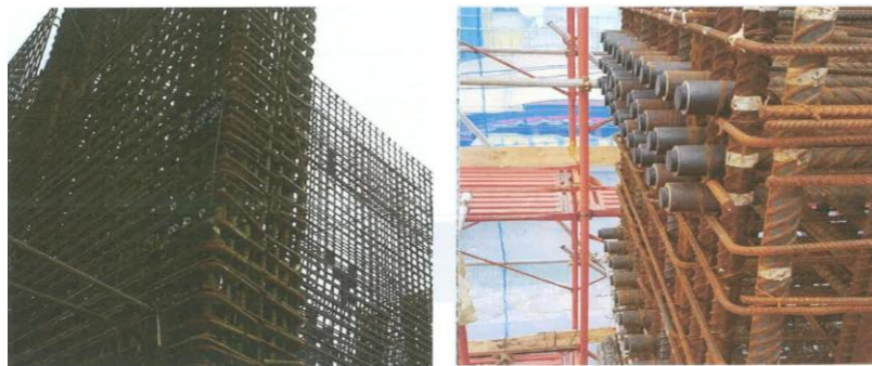
Gambar 6. Joint Rebar Coupler
